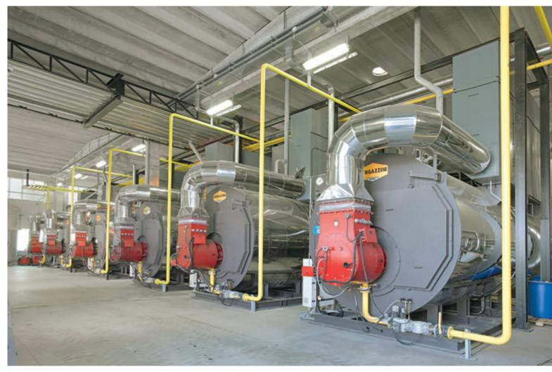
▲ Turn-key boiler room, composed of n. 6 steam boilers mod. PB 200, equipped with energy recovery system, steam output of each boiler: 20,000 kg/h.
