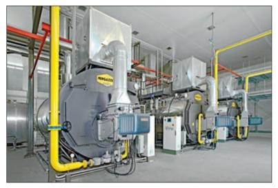
▲ Turn-key boiler room, composed of n. 3 steam boilers mod. PB 120, equipped with energy recovery system, steam output of each boiler: 12,000 kg/h.
