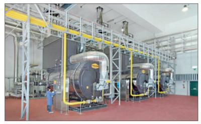
▲ Turn-key boiler room, composed of n. 3 steam boilers mod. PB 120, equipped with energy recovery system, steam output of each boiler: 12,000 kg/h.
