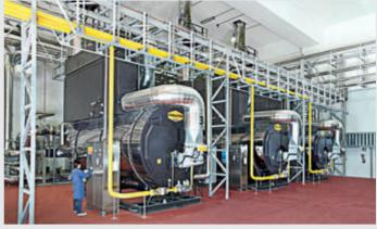
$\blacktriangle$  Turn-key boiler room, composed of n. 3 steam boilers mod. PB 120, equipped with comburent air preheater, steam output of each boiler: 12,000 kg/h.
